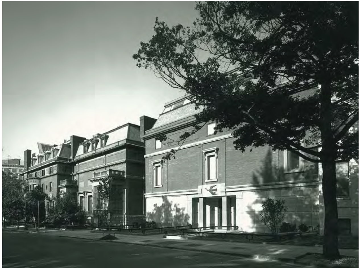
The House and Goh Annex, 1989
